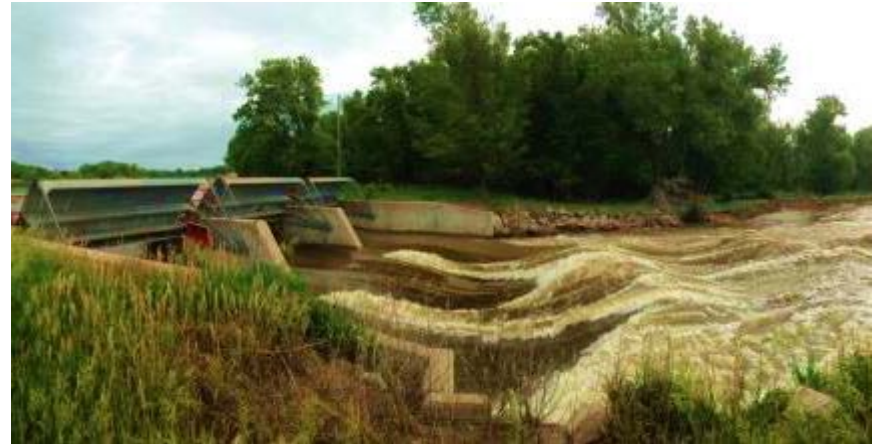
30-Mile Canal Headworks, June 2015
